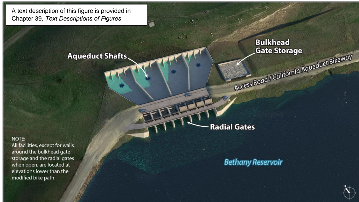
5 6 Figure 3-34. Bethany Reservoir Discharge Structure
