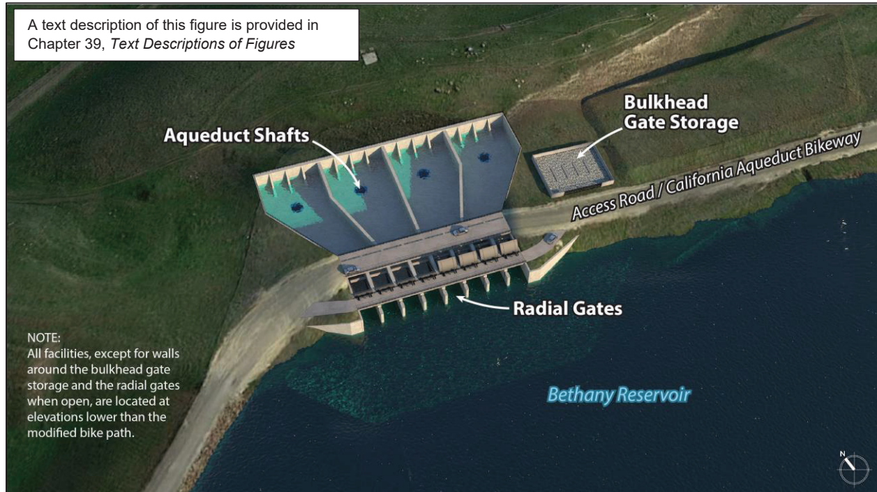
5 6 Figure 3-34. Bethany Reservoir Discharge Structure
