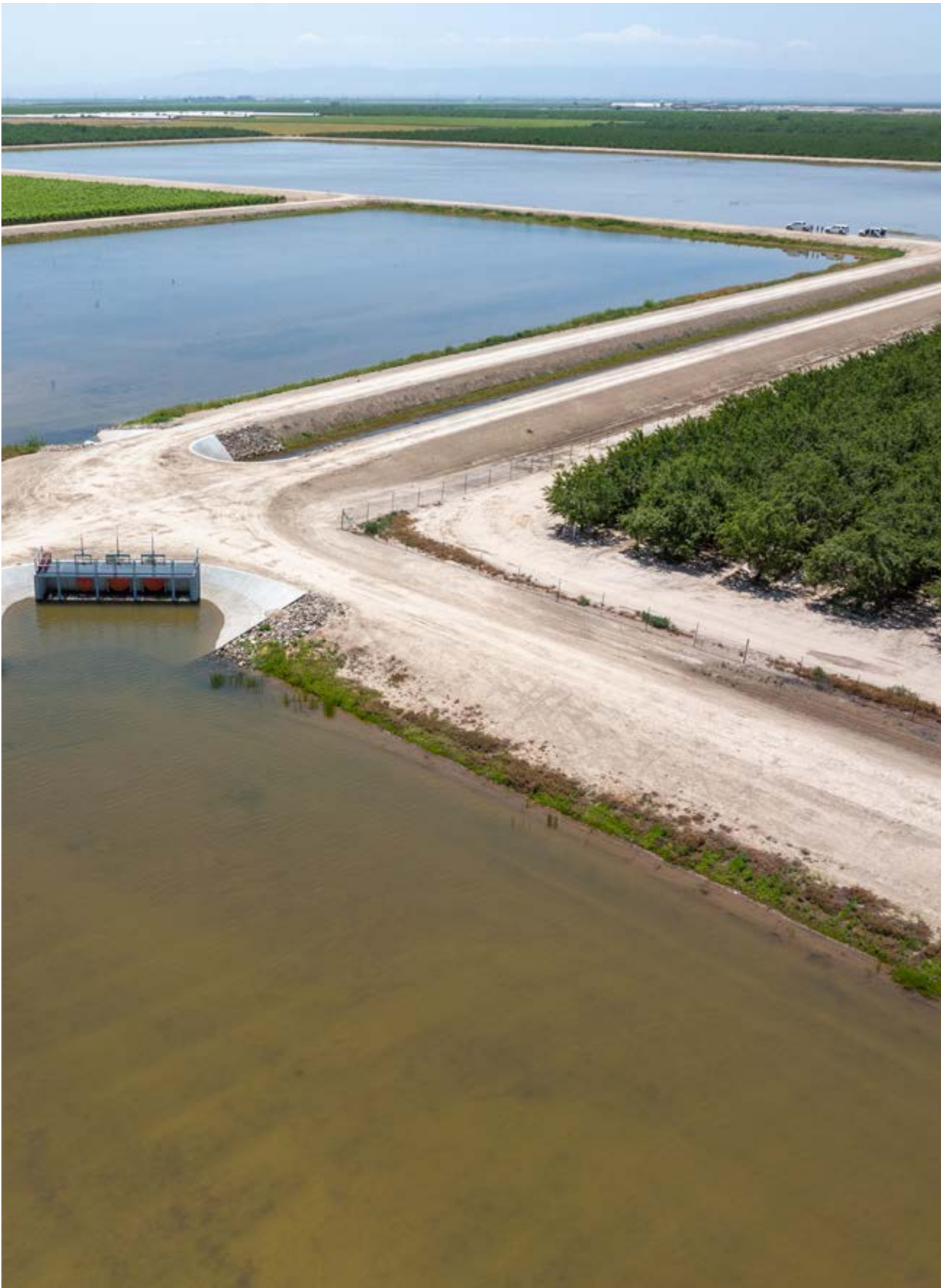
California Department of Water Resources, Statewide Infrastructure Investigations Branch
