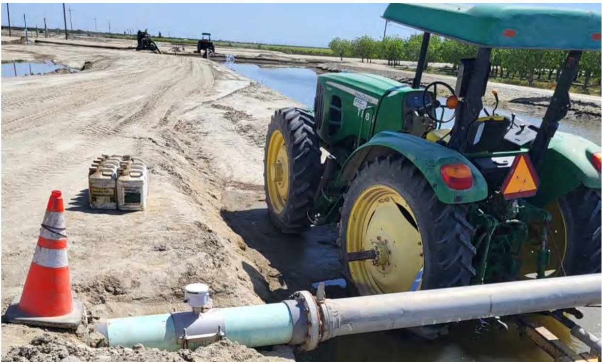
Water metered and pumped from internal canal into a pistachio orchard.
