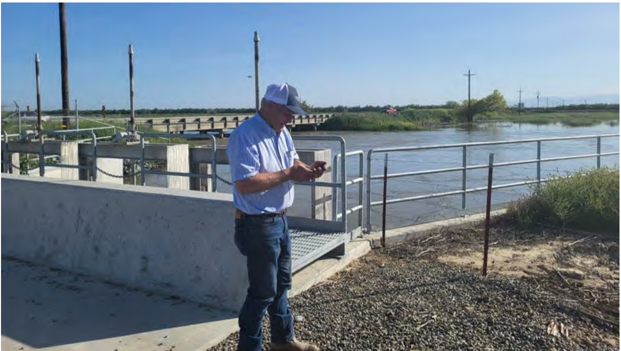
Mr. Cameron, using his computer telemetry to control the height of the turnout flood gates.
